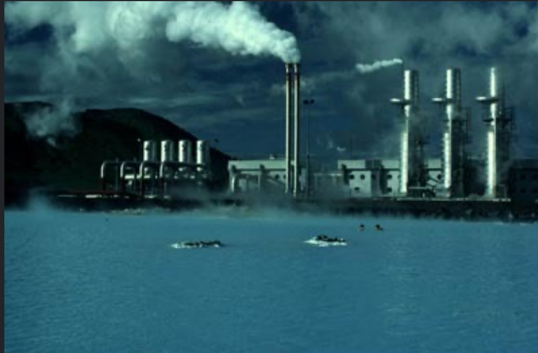
Geothermal energy plant in Iceland
