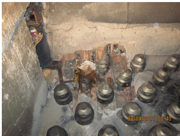
Gambar 2.23 Inspeksi Fluidizing Air Nozzle
