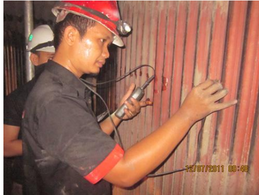
Gambar 2.54 Thickness test Tube Boiler
