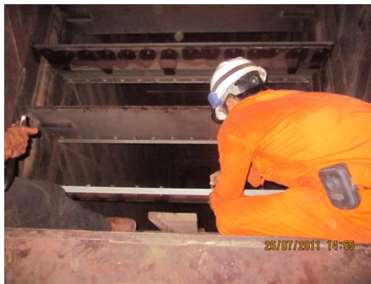
Gambar 2.14 Inspeksi discharge damper
