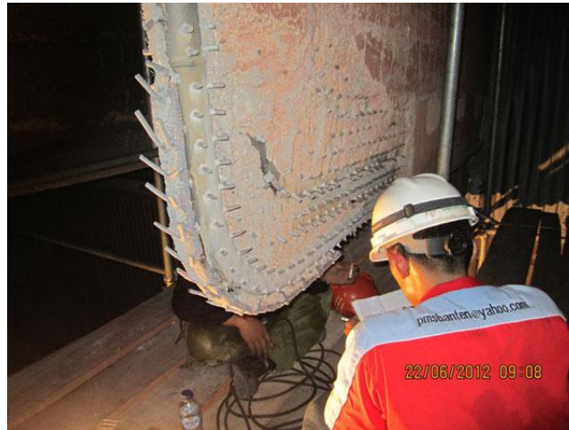
Gambar 2.22 Inspeksi Tube & Refractory Wingwall (Evaporator panel)
